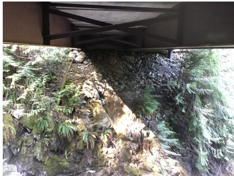
Left Bank Abutment when facing downstream
