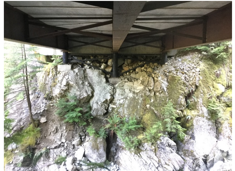
Right Bank Abutment when facing downstream
