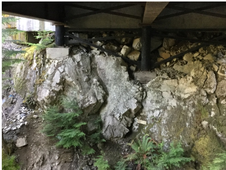
Right Bank Abutment when facing downstream
