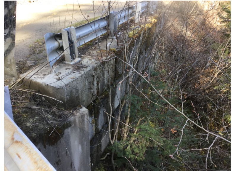
Downstream left bank wingwall
